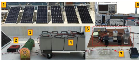
1. PV panels 2. MPPT 3. Resistive load 4. Batteries 5. Oscilloscope, amplifiers and sourcemeter 6. Arc generator 7. TMR 2001
